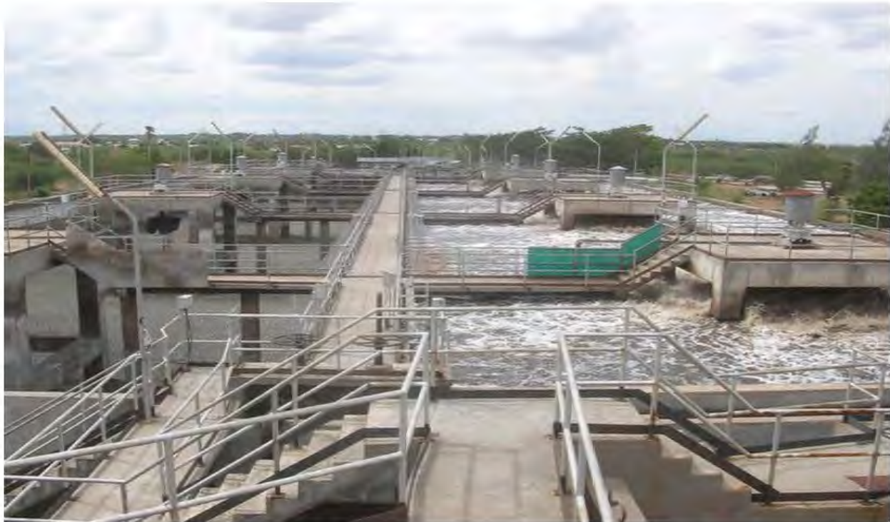
View of Existing STP
